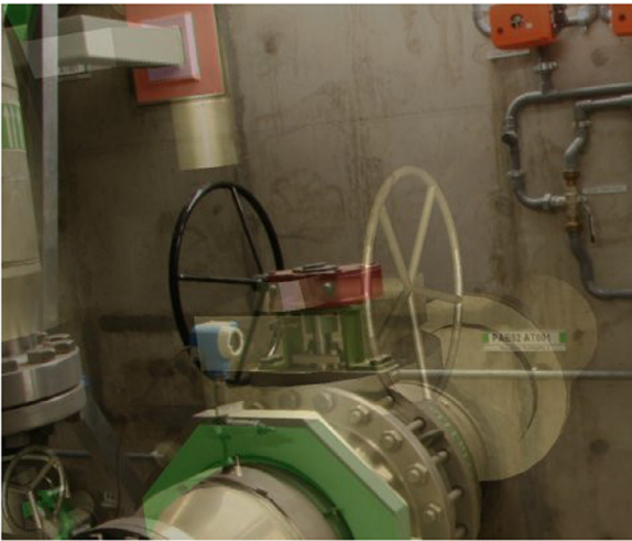
Fig. 4. Example of inspection task using AR (Georgel et al., 2007).
