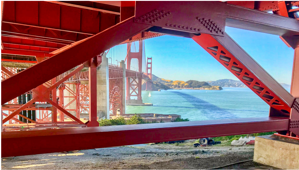
Figure 2.2 View from underneath the Golden Gate Bridge showing its truss structures.
